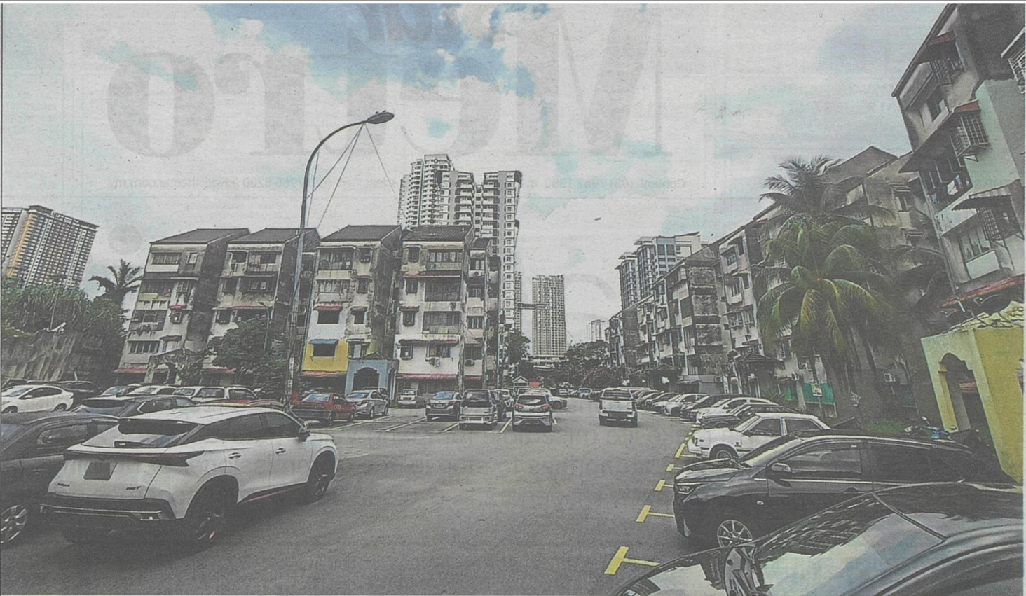
Ongoing management issues at Flat Taman Kobena in Cheras, Kuala Lumpur, have plagued building maintenance since 1995.
